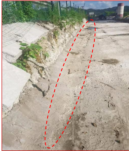
(a) 衔接面处砂浆封闭
